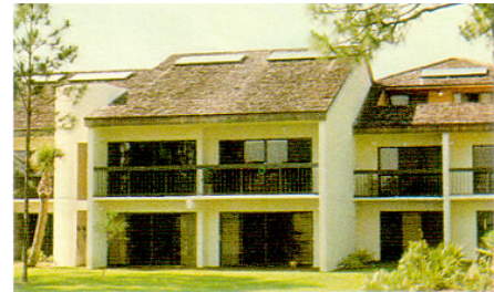
Sunstar Collectors on new construction designed to look like skylights.
